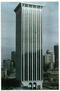
Fig. 6. Dalian Xiwang Building, Dalian City, China. The table below shows substantial savings in concrete and steel quantities by using precast/prestressed concrete technology. This building is located in a high seismic zone and, therefore, savings in materials will result in lower building dead weight and subsequently lower shear forces due to seismic loads.
